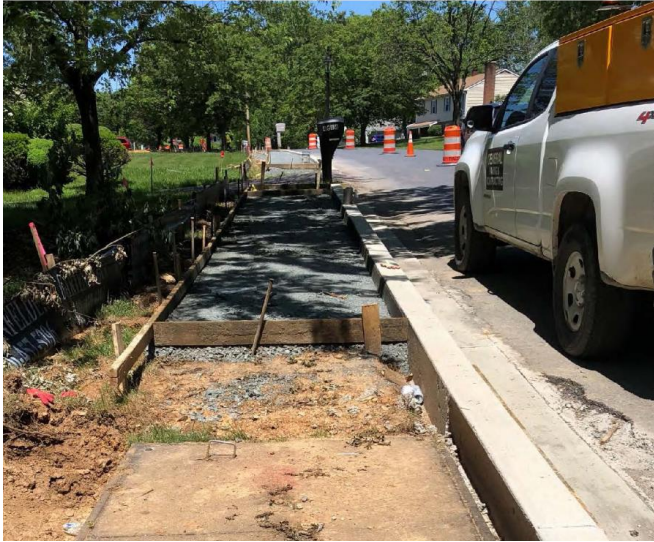
Sidewalks being replaced.
